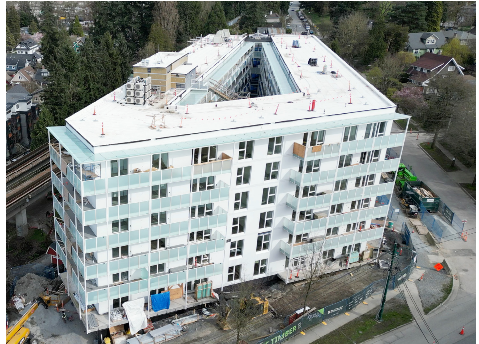
Vienna House, Vancouver under construction. Vienna House used BIM during design and construction, and is providing asset data for FMO. (photo: Bright Future Studios)
